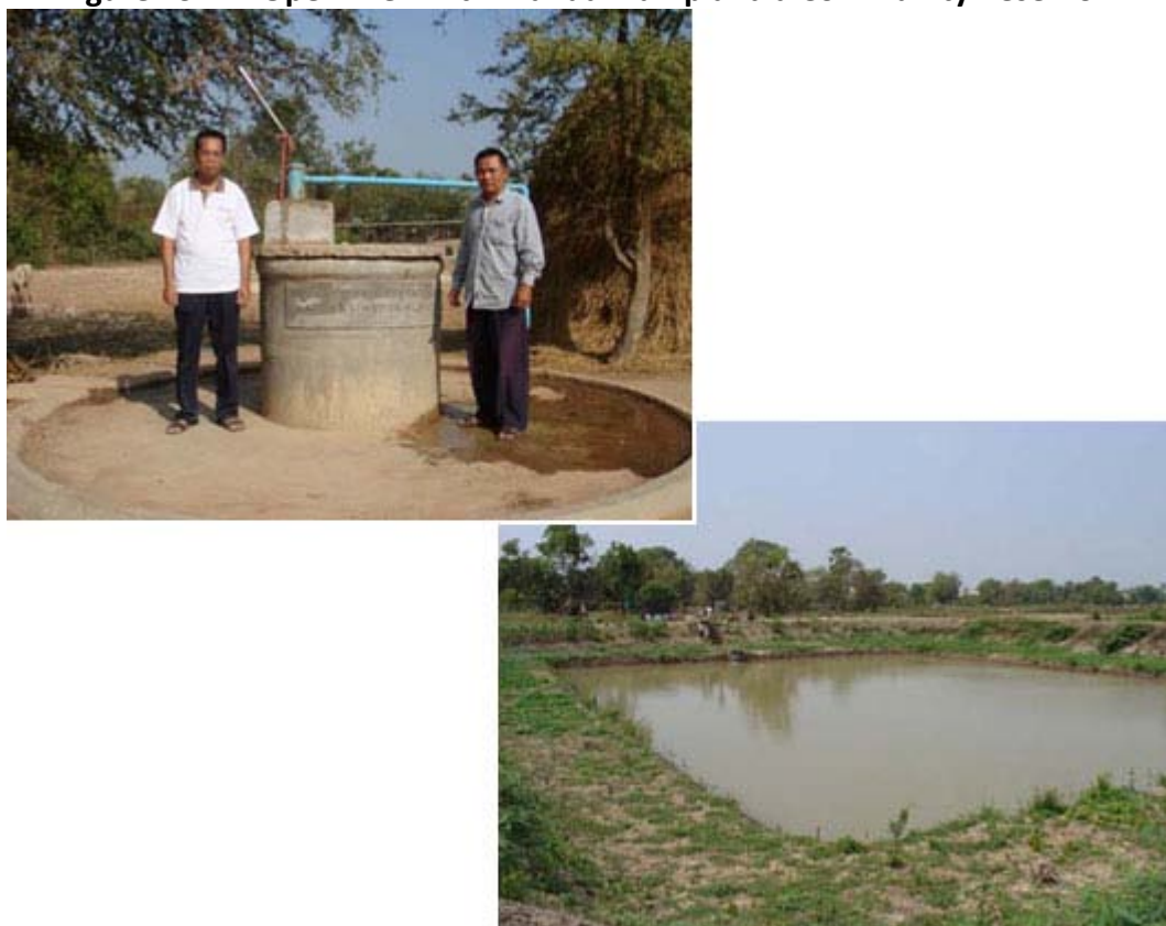
Figure 13: An Open Well with Manual Pump and a Community Reservoir
