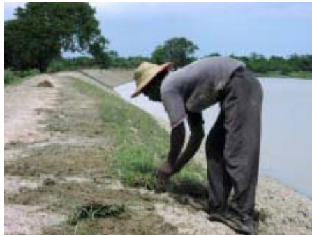
Turfing against erosion (5)
