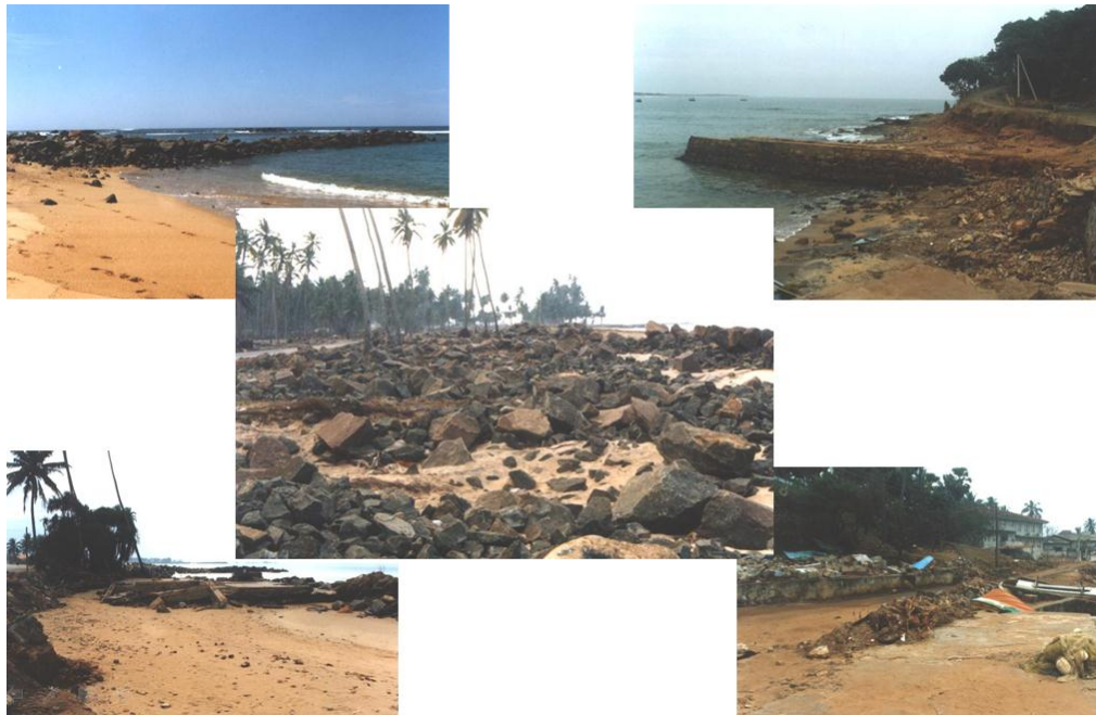
Plate 1: Disturbed revetments & groins in the Southern Coastal belt of Sri Lanka during tsunami
