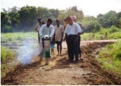
Compacting the bund (5)
