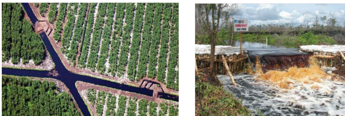
Figure A-2 Water management technology: comb structures applied to HTI drainage channel at Kampar Peninsula, Riau (left) and Tabat (right) applied to agriculture land rehabilitation in central Kalimantan (Hooijer at al, 2007)
