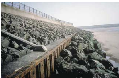
An example of revetment (Source: http://www.snh.org.uk/publications/on-line/heritagemanagement/erosion/appendix_1.16.shtml )
