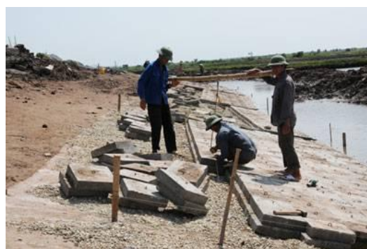
Figure 11 - Dyke reinforcement in Thuy Hai, Thai Binh
