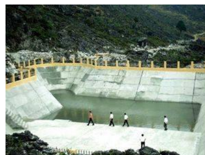
Figure 14 - A water-collecting reservoir in Ha Giang
