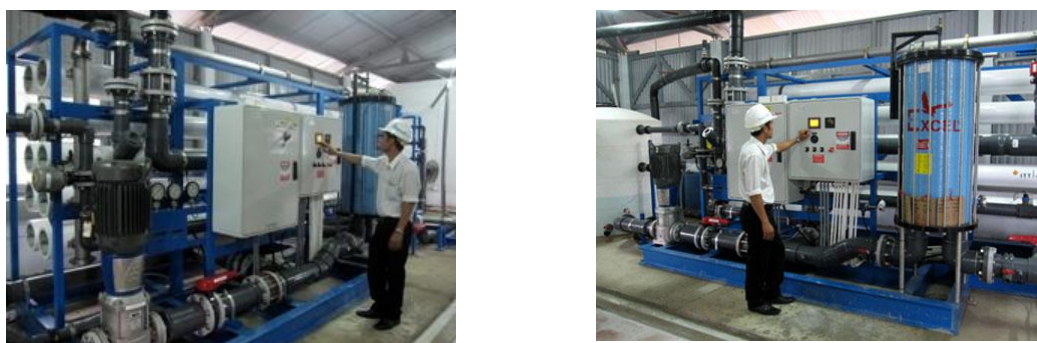
Figure 15 - Desalination system in Vinpearl Land tourism and recreation area on Hon Tre Island
