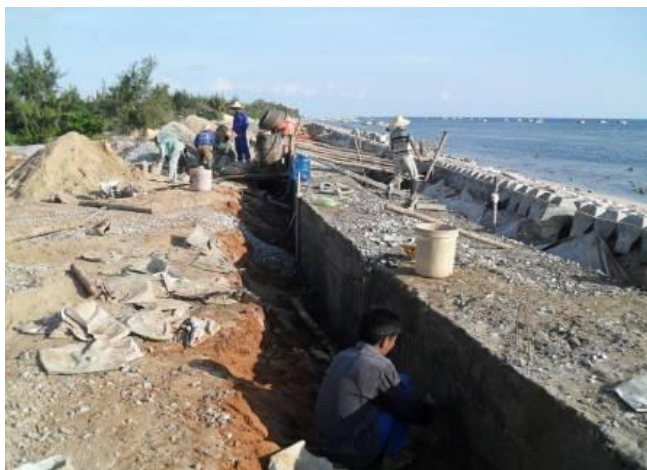
Figure 12 - construction in Phu Quy Island
